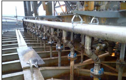
SS PIPE MANIFOLD
