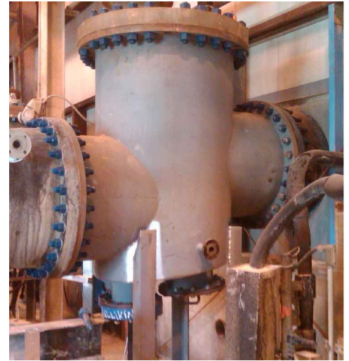
Hastelloy Lined Strainer Housing
